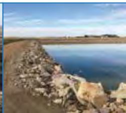
Waste Water Management
