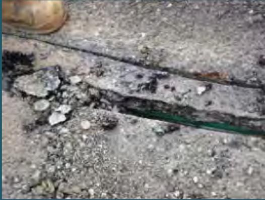
The fibre-optic cable is placed into the micro-trench along with a tracing cable.
