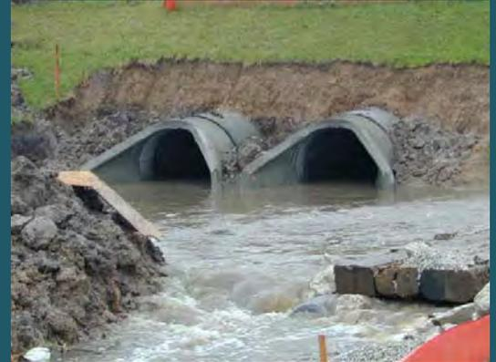
The picture below, by Russell Humphrys, reproduced from Najafi et al, 2005, shows the emerged leading end of a pipe installed in an evaluation project using the open-faced pipe ramming technique. Note the reinforced leading edge of the pipe, and bentonite feed line at the top of the pipe.
