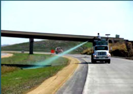
The picture below, courtesy of Nilex Inc., shows the installation of MulchMax hydraulic mulch, which allows the simultaneous application of seed and mulch. See Appendix 7 for MulchMax Installation Guide.
