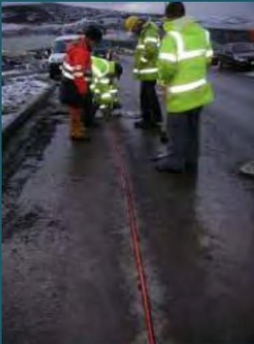
The trench is backfilled with a suitable crack sealant.
