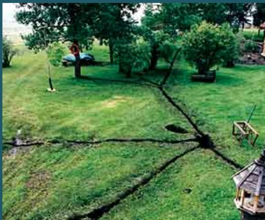
In wintertime, excavating frozen ground using a backhoe can pose a number of challenges. Hydrovac technology offers an alternative solution. It consists of slot-trenching the excavation area (which is cleared of asphalt pavement in advance using a saw) in a grid pattern, then “plucking” the frozen cubes of soil. The technology should not be used around buried utilities, which should be hydrovaced by traditional methods in advance (Coburn, L., 2012).
