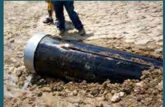
The picture below, by Chris Wilke, shows the installation of a culvert on Provincial Highway No. 1 near its intersection with Lewvan Dr. in Regina, Saskatchewan, using the open-faced ramming method. Note the auger used to remove the soil inside the pipe. Picture courtesy of Clifton Associates Ltd., 2011.
