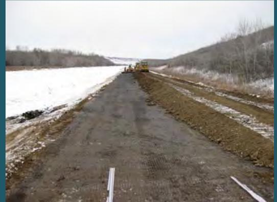
Geo-grids such as in the picture above have significant lateral and longitudinal tensile strength, while its structure allows interlocking with the granular material which keys it into place. Geo-grids can be used over extended road lengths or in localized spots, such as trench cuts, where subgrade and moisture conditions negatively impact the road's performance.
