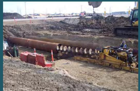
The four pictures below, by Grant Gilliss, courtesy of Clifton Associates Ltd., show the installation of a water pipe over 1 km length using the “boring” method. The entry and exit points of the pipe are excavated, then a boring machine drives the cutting head in, followed by the pipe. The maximum length over which the pipe can be driven from one end is limited by the equipment driving pressure; however, technological advancement is continuously increasing this limit.
